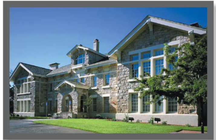
St. Helena High School, built in 1912, is recognized in the National Register of Historic Places in Napa County
